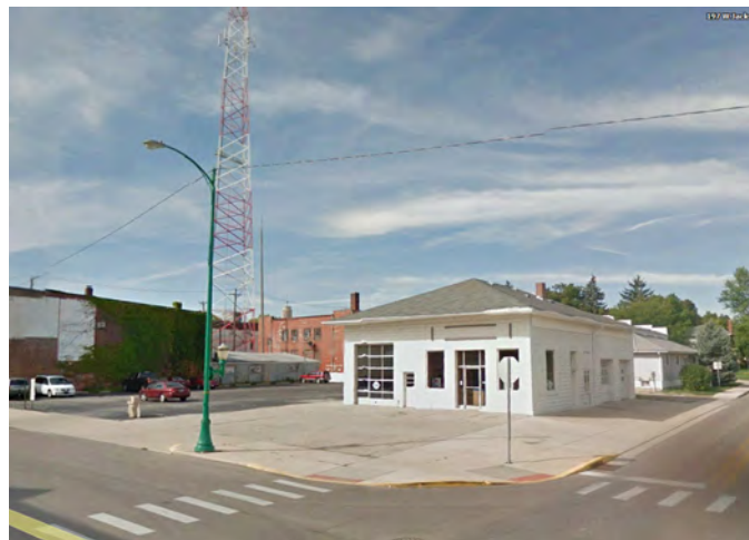
The corner lot transitions from commercial to the south and residential to the north. The incorporation of landscaping along the streetscape would blend the transition, as well as provide safety for pedestrians. Pedestrian and vehicular traffic should be separated on the site and identified through the use of different materials and landscaping. The corner lot also allows for the opportunity for additional streetscape amenities, such as sculpture and benches.
