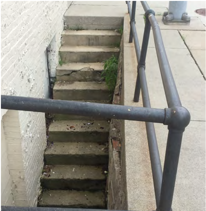
Located on the west side of 144 West Monroe, this exterior stairwell is significantly deteriorated and in need of immediate repair or enclosure.
