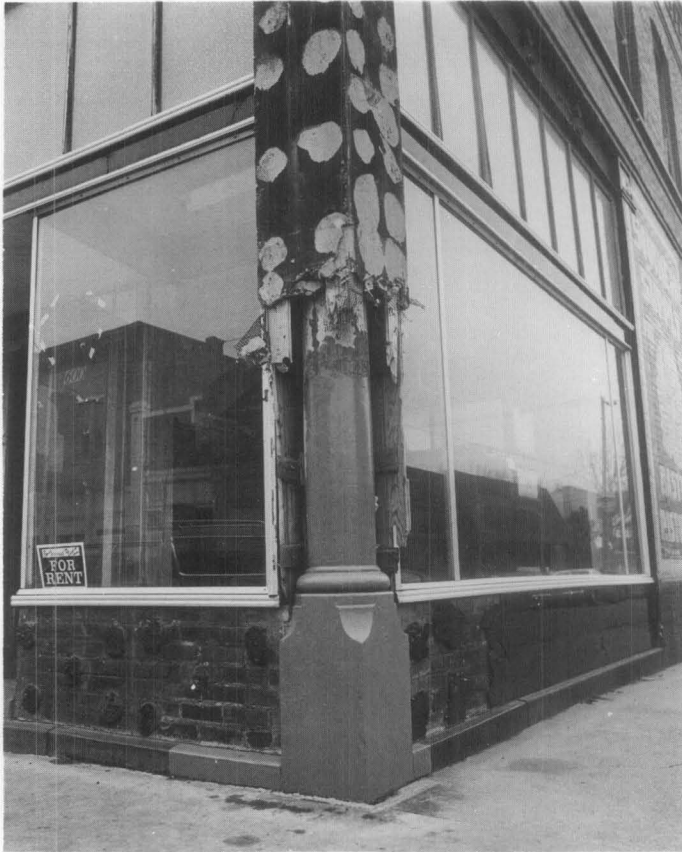
Figure 6. Storefronts of the 1940's, 50's, and 60's were frequently installed by attaching studs or a metal grid over an early front and applying new covering materials. If the existing storefront is a relatively recent addition with little or no architectural merit, begin by removing the covering materials in several places as was done here. If this preliminary investigation reveals evidence of an earlier front, such as this cast-iron column, carefully remove the later materials to assess the overall condition of the historic storefront. The black mastic visible on the lower masonry panels was used for installing pigmented structural glass. Some attachment methods for modern facings, such as mastic or metal lath, may have seriously damaged the original fabric of the building, and this must be taken into account in the rehabilitation process. Photo: Bob Dunn
