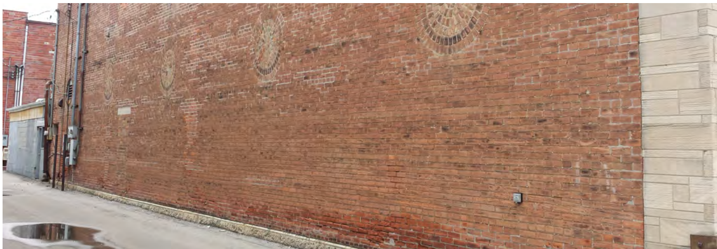
Tuckpointing is needed on the upper facade. The paint should be removed from the brick. The cornice detail should be repaired and painted in a historical color to coordinate with the building, while the glass block windows should be replaced with windows in keeping with the original style.
