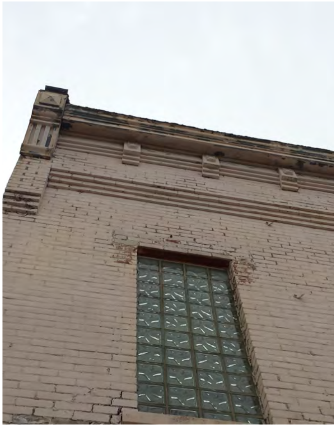
Tuckpointing is needed on the upper facade. The paint should be removed from the brick. The cornice detail should be repaired and painted in a historical color to coordinate with the building, while the glass block windows should be replaced with windows in keeping with the original style.
