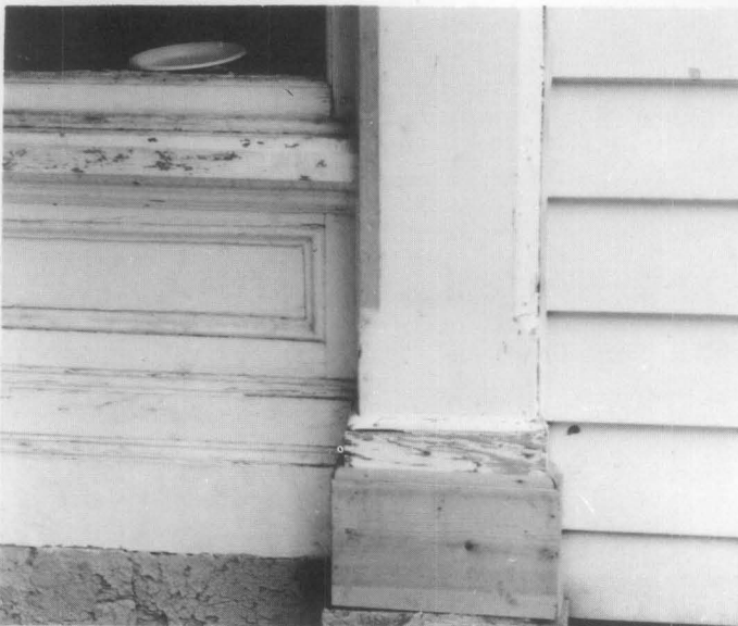
Figure 9. Rather than replace an entire wooden storefront when there is only localized deterioration, a new wooden component can be pieced-in, as seen here in this column base. The new wood will need to be given primer and top coats of a high quality exterior paint—either an oil-base or latex system. Also wood that is flaking and peeling should be scraped and hand-sanded prior to repainting. Photo: H. Ward Jandl
