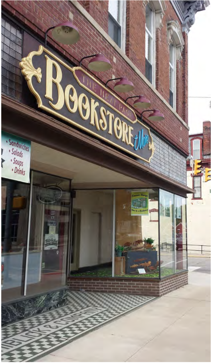
The above image shows an excellent example of an appropriate cornice, upper facade, transom, storefront windows, and bulkhead.
