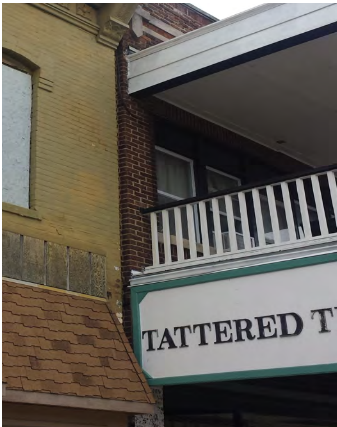
Infilled transom window.
