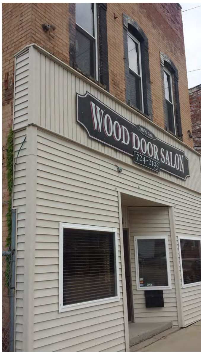
A closeup view of the storefront system.
