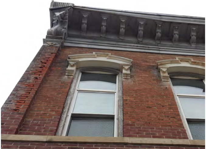
The upper facade has areas that need to be tuckpointed and caulked, and trim needs to be painted. The cornice needs some repairs and paint as well.
